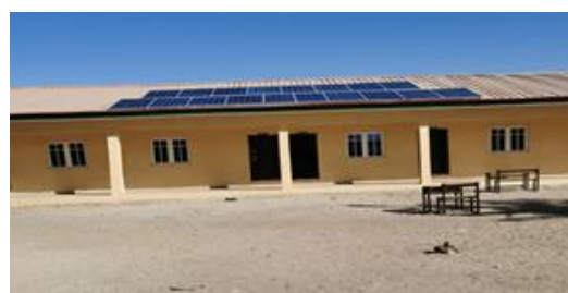
5 KVA solar power installed at Mafa School, March 2021 (Photo: UNDP)
