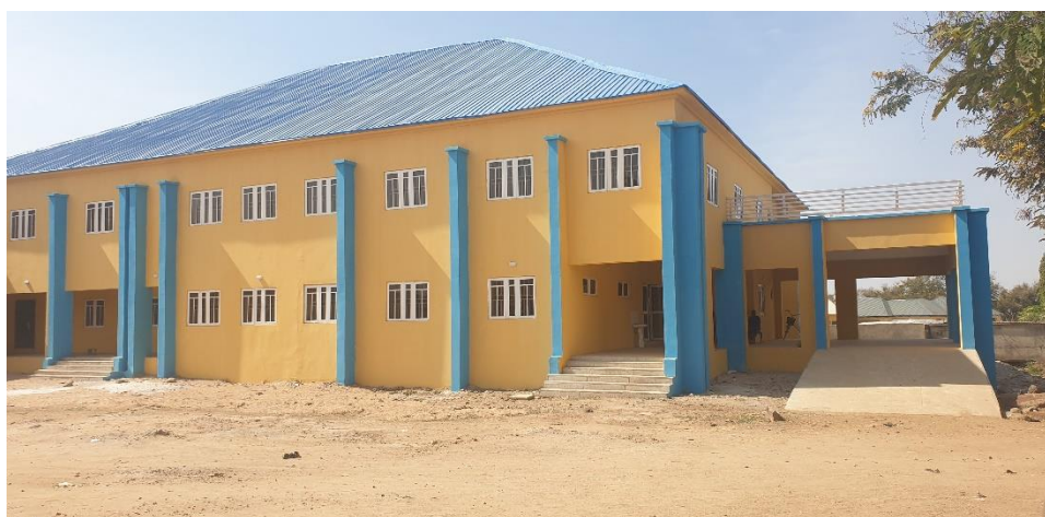
Completed Biu General Hospital (Phase 2)
